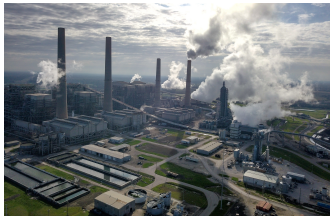
Coal-fired power plant: Petra Nova
